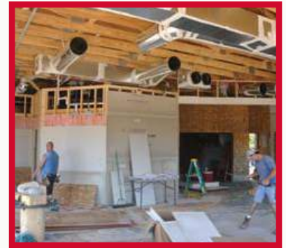
Installation of dry wall begins.
